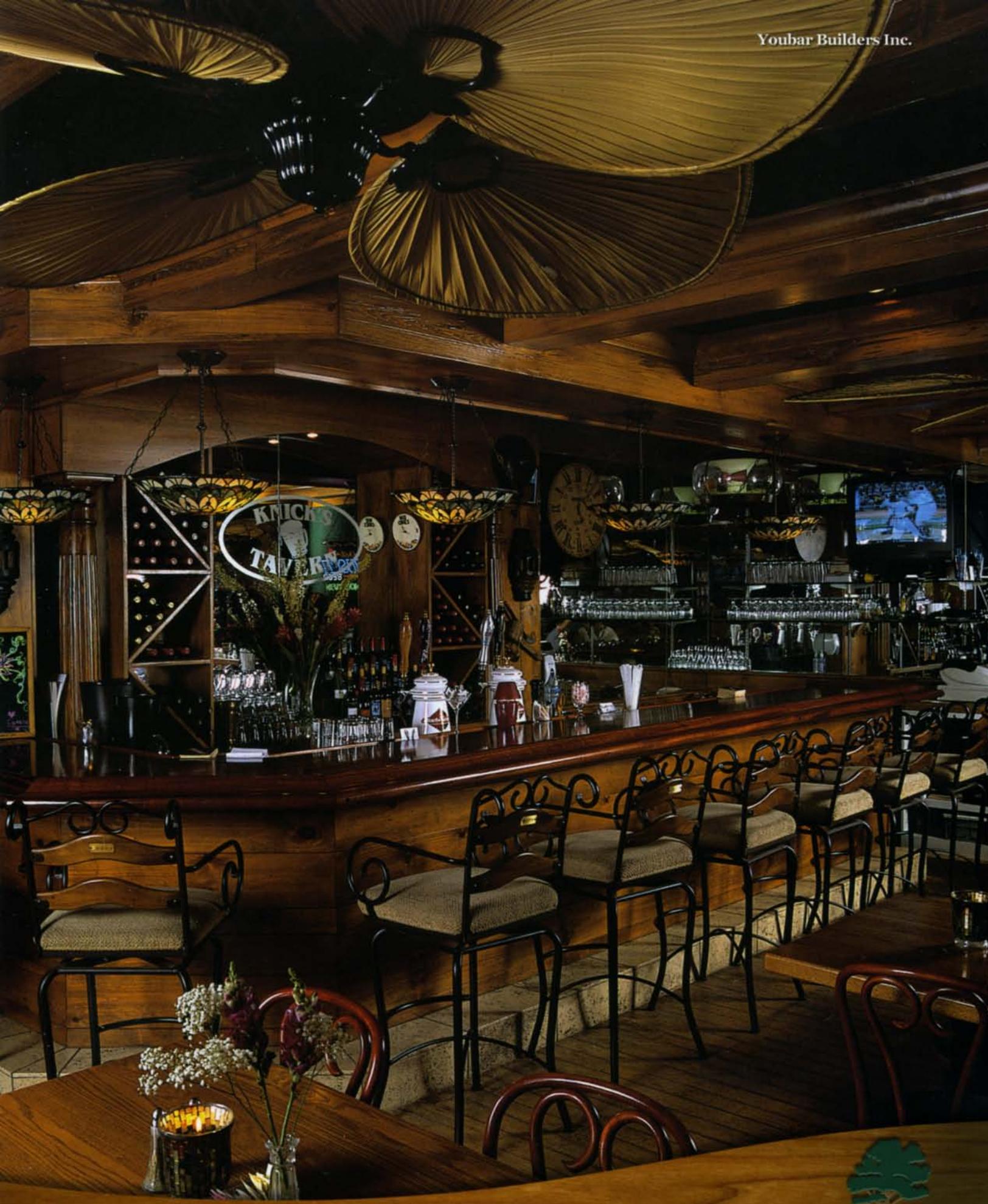
Pecky Cypress Beams, Crown, Soffit, Goncalo Alves Bar Top and Rail, T & G Paneling, Bamboo Flooring, Solid Oak Tabletops
